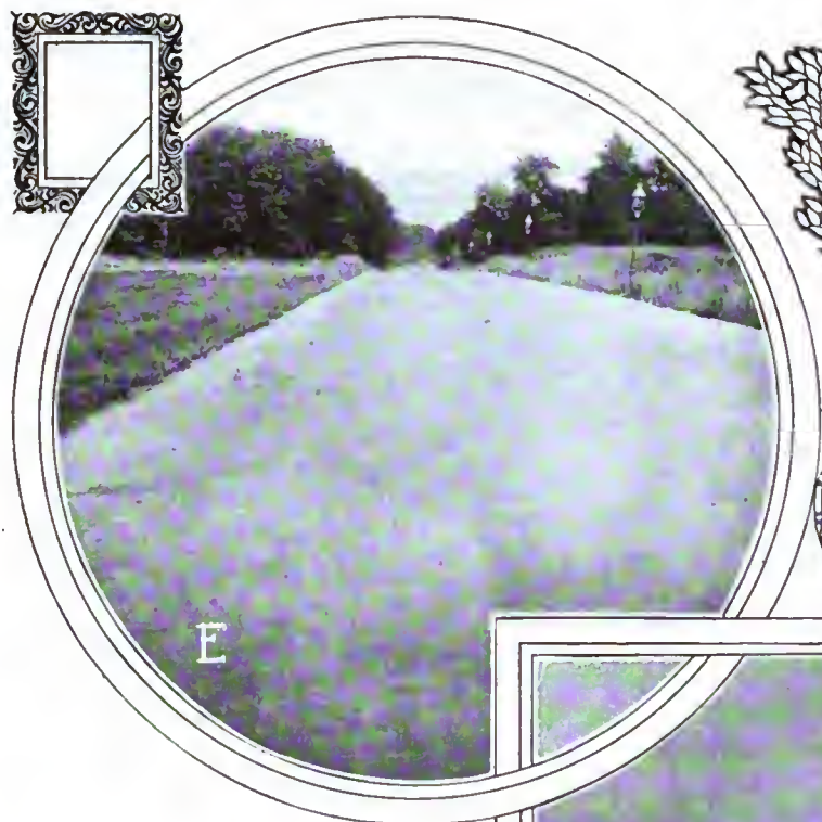
E—General view of the cement block road adjoining the Pelham Parkway, in which the good even surface will be noticed
